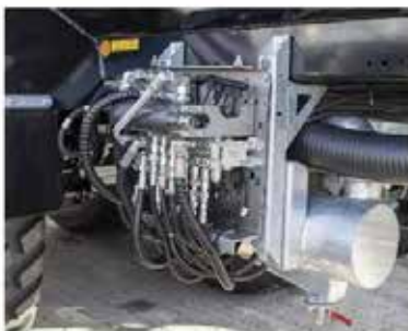
Hydraulic control block
